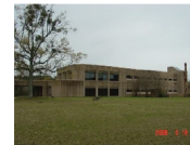
TRAVIS CLINIC BUILDING
